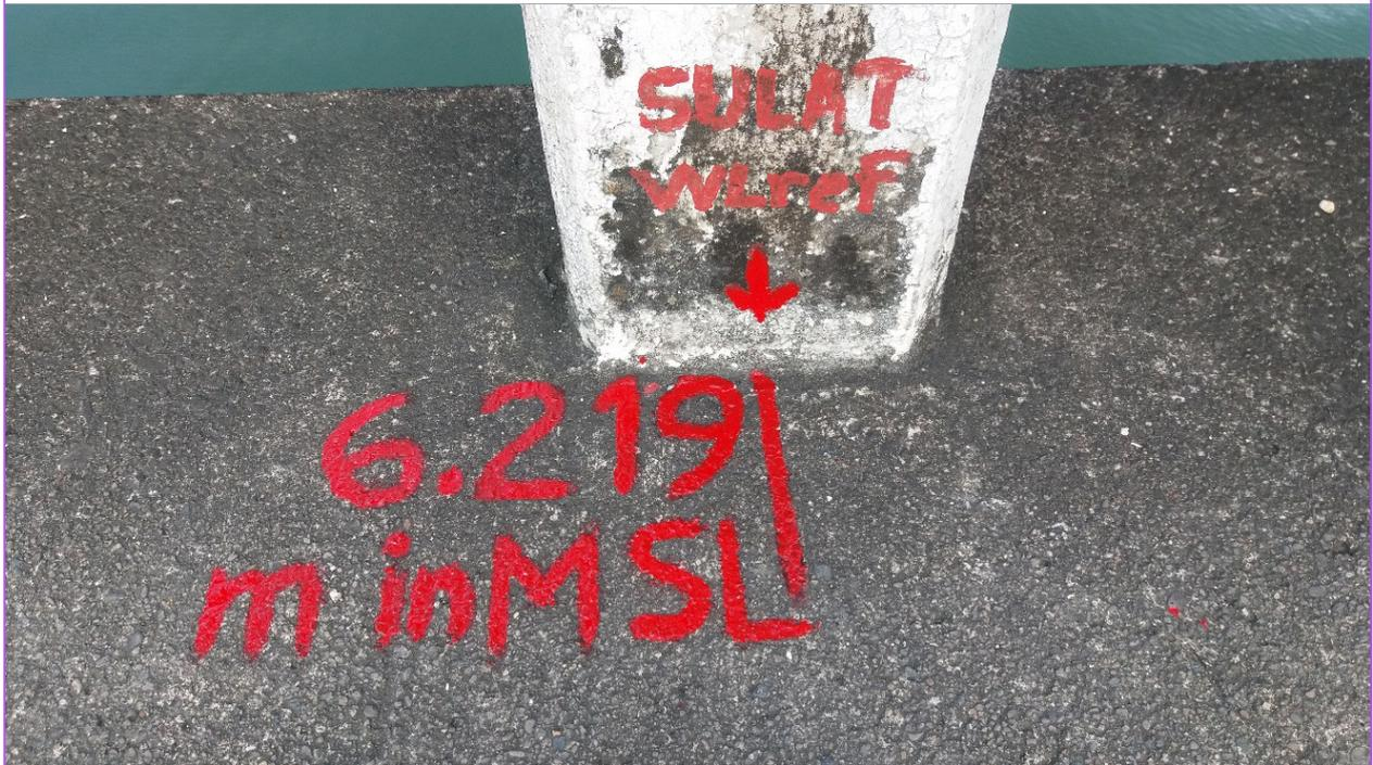
Figure 41. Water-level markings on Sulat Bridge.
