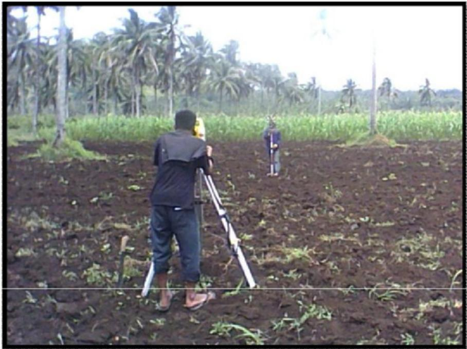
**Figure 16.** Conducting cross-section survey using Hi-Target Prism less at cross-section 12 at Brgy. Matampay, Baloi
