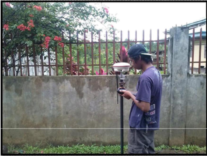
Figure 17. Conducting cross-section survey using RTK at cross-section 8 at Brgy. Poblacion, West, Baloi
