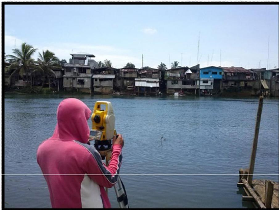
**Figure 21.** Conducting profile survey using Hi-Target Prism less at Brgy. Poblacion West, Baloi
