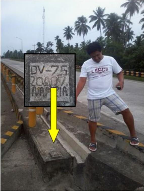
Figure 35. Static GPS observation in DV-75 which is 100 m away from KM 1468 post along the national highway at Barangay Guadalupe, City of Carmen
