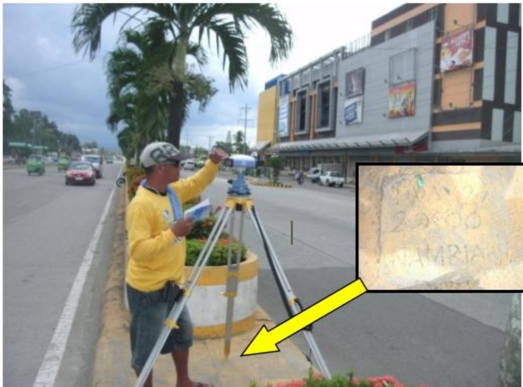
**Figure 33.** Static GPS observation in DVA-12 at the center island in front of CENRO office
