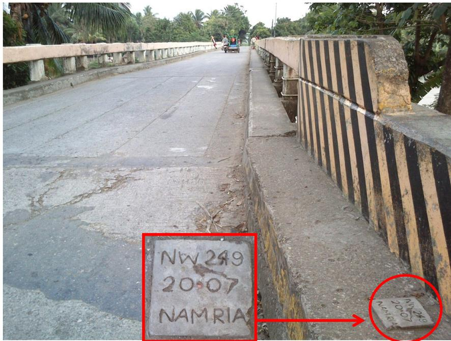
**Figure 13.** NW-249 located at Sitio Malabong, Malabong Bridge considered as a ground control point for the creation of GNSS Network
