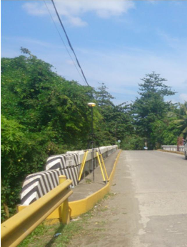
Figure 12. Static GNSS observation at control point at Lanag Bridge 1 in Sta. Barbara
