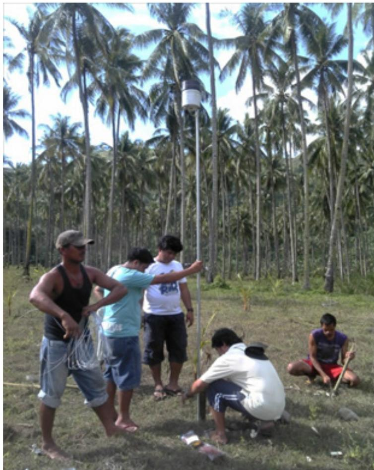
**Figure 23.** Rain Gauge installation in Brgy. Sta. Ines, Malitbog, Bukidnon
