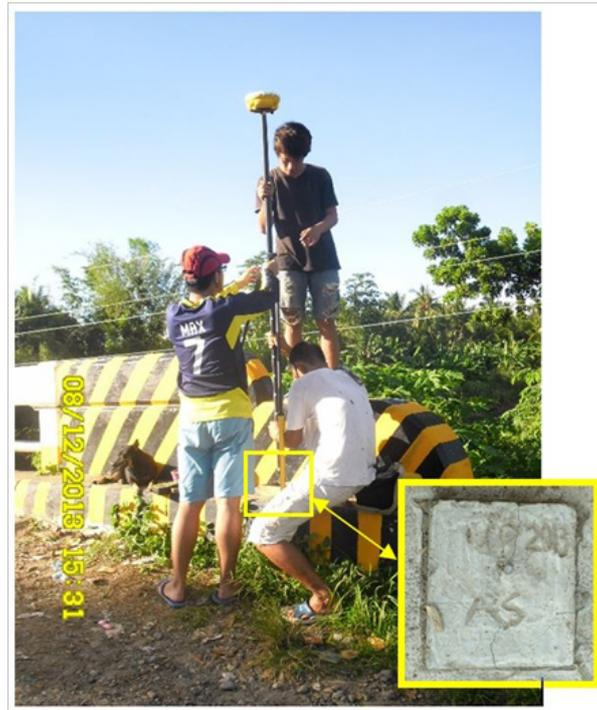
**Figure 16.** Static GNSS observation at UP-AS in Brgy. Poblacion, Asuncion
